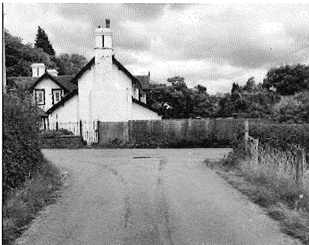
Figure 5: showing the entrance from Stoney Low onto Three Mile Lane, indicating the poor visibility.
